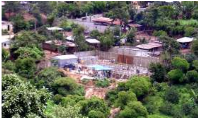
Feeding Center Construction seen from the road above
