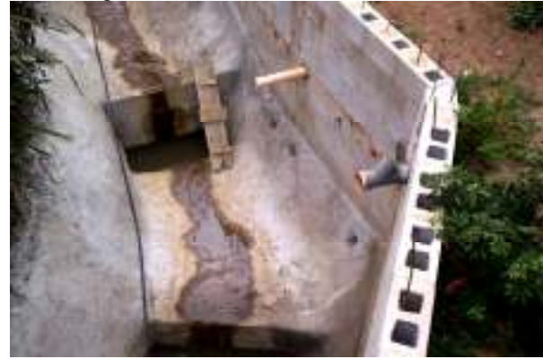
Barranco turned into a concrete drainage channel
